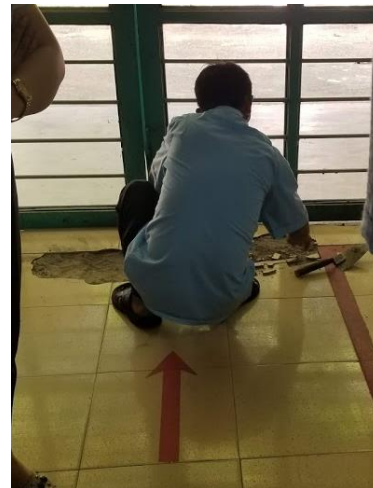
Figure 6: Employee Repairing Broken Flooring
