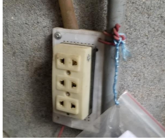
Figures 29 and 30: Ungrounded Electrical Outlet in Fire Pump Room
