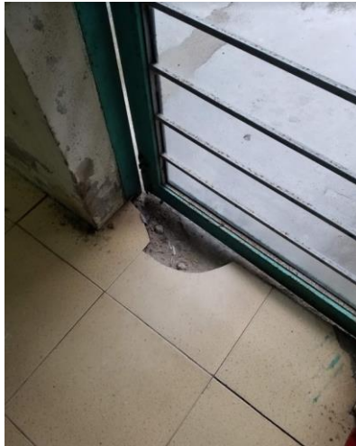
Figures 4 – 5: Broken Flooring at Exit Doorway
