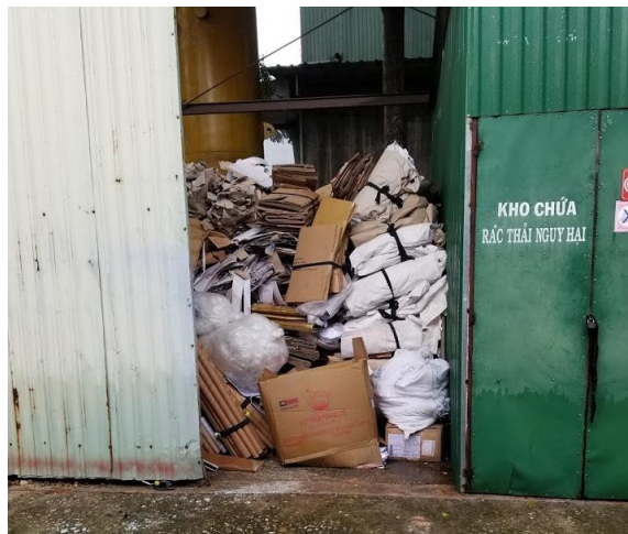
Figure 7: Overflowing Combustible Waste Storage next to Hazardous Waste Storage (“Kho Chứa Rác Thái Nguy Hại”) Area.
