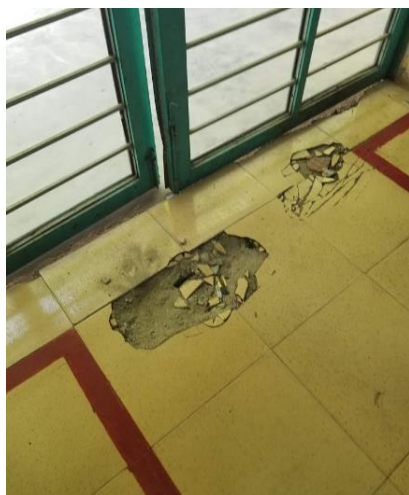
Figures 4 – 5: Broken Flooring at Exit Doorway
