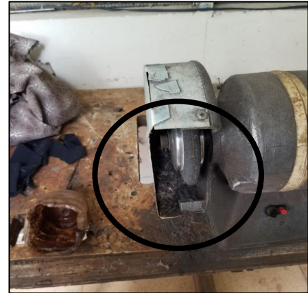
Figure 19: Unshielded Grinding Wheel
